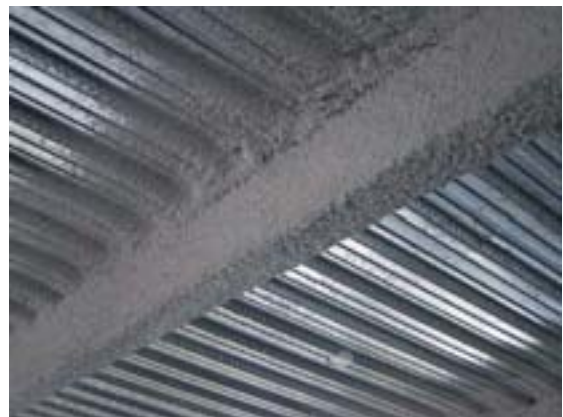
Fig I.1 Beam protected with SFRM.
