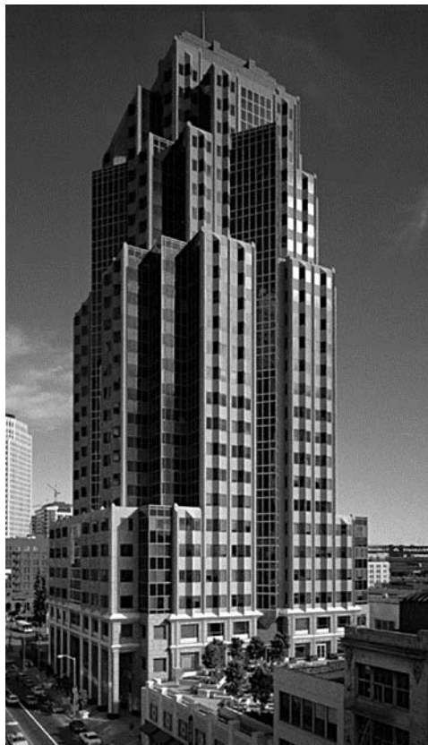
Figure 1. First Street Plaza Building Constructed with Braced Frames and CFT Columns
