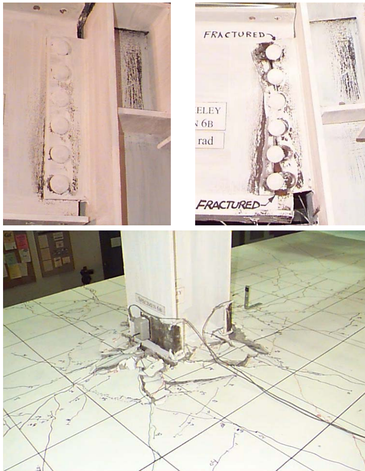
Figure 4. (Clockwise from Top Left) 6-bolt Shear Tab Connection with Slab (6B) at 0.03 Radians, Connection at 0.11 Radians (End of Test), Floor Slab at End of Test
