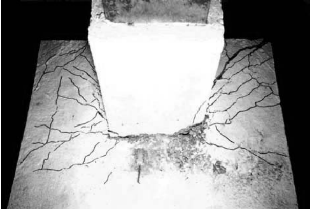
Figure 11 - Hysteresis loops and failure mode of an external node with a composite column.
