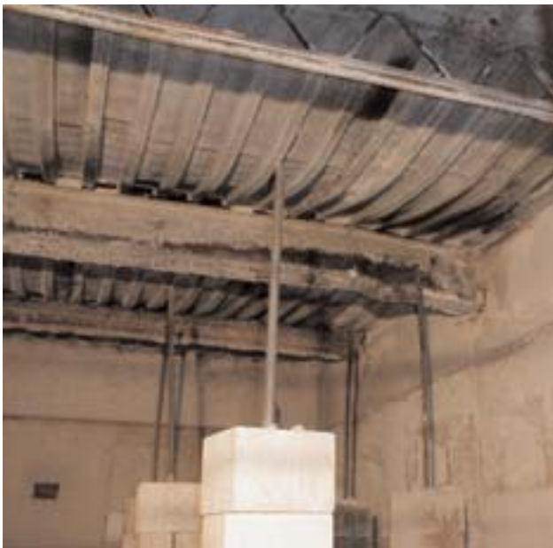
Fig. 6.1. UL Steel Roof Assembly After Successful ASTM E119 Fire Test (Courtesy of Underwriters Laboratories, Inc.)
