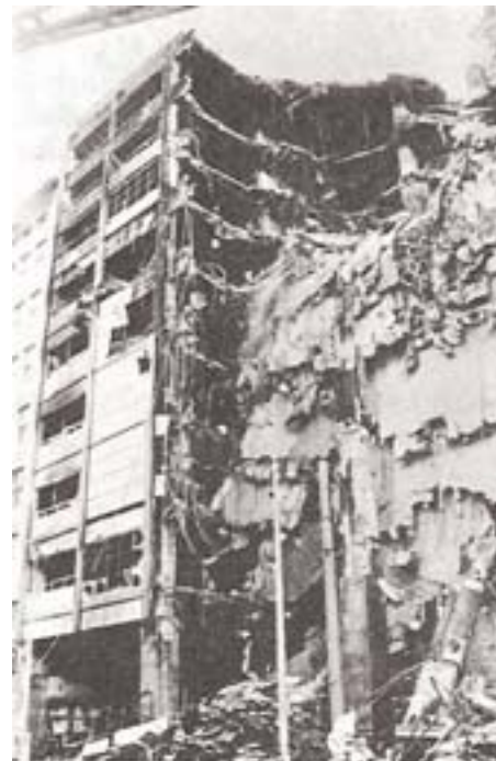
Fig. 7.3. Katrantzos Department Building in Athens, Greece, After 1980 Fire (Papaioanna, 1986)
