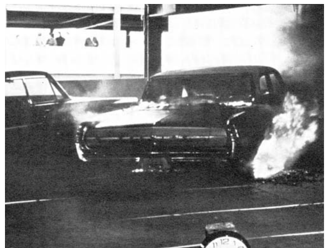
Fig. 8.1. Burning Automobile After 24 Minutes in 1972 Scranton Fire Test of Parking Garage (Gewain, 1973) ( Modern Steel Construction , 1973)
